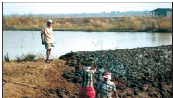
Fig. 8 : Pitching of bund with black clayey soil
